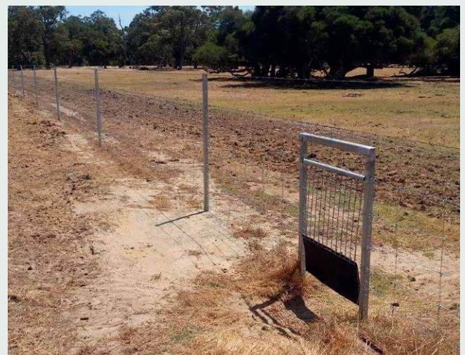
Kangaroo gate provides safe access across landscapes.
